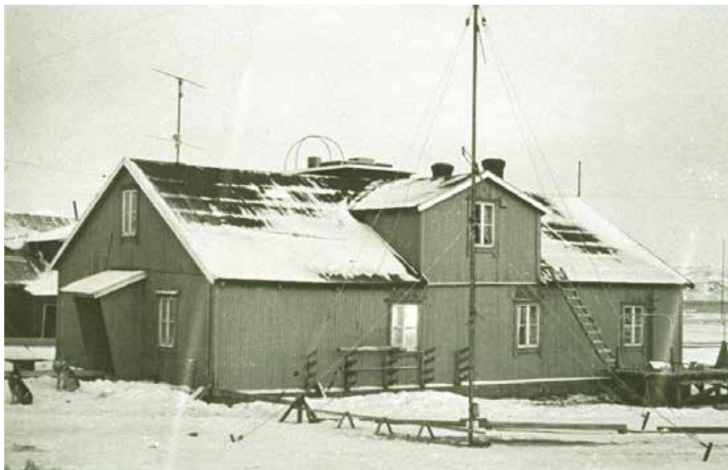
The first research station 6 in Ny-Ålesund came in 1966-67. It had instrument platforms on the roof and on the ground. Offices for the scientist were on the ground floor.
