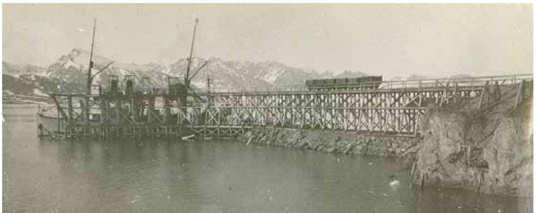
The coal quay in 1925. Today's quay is here 53 . On the quay we can see coal wagons. A ship is being loaded through coal shuts. Photo: Helge Hjelle, Norwegian Polar Institute.
